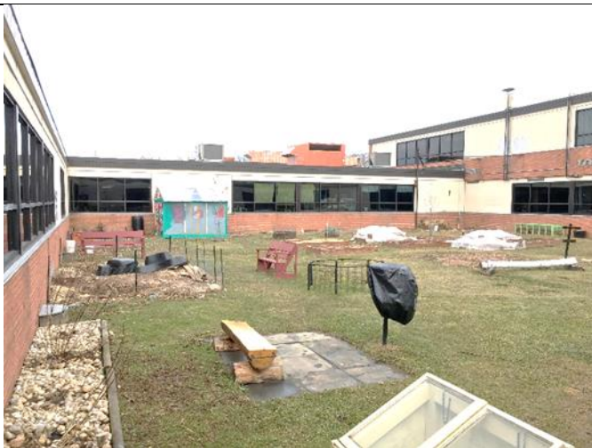
EIFS 5 First Floor HS (courtyard)
