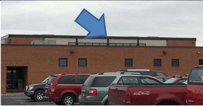
EIFS 6 Old Gym Upper Level (Gable 4)
